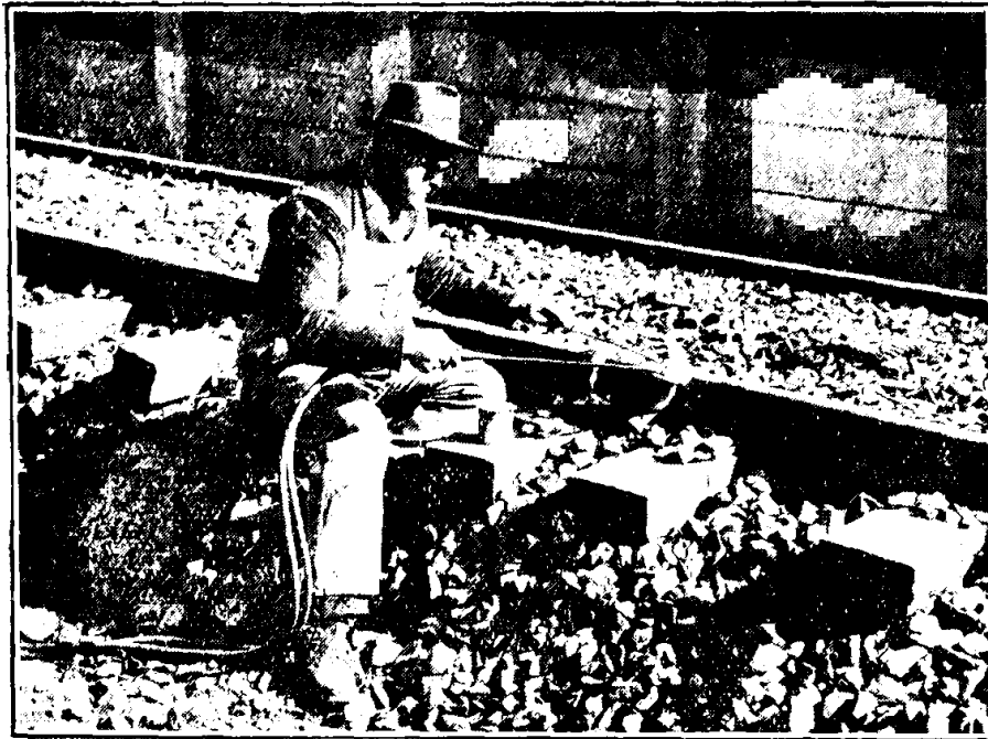
Fig. 13.—Rail Bonding.
