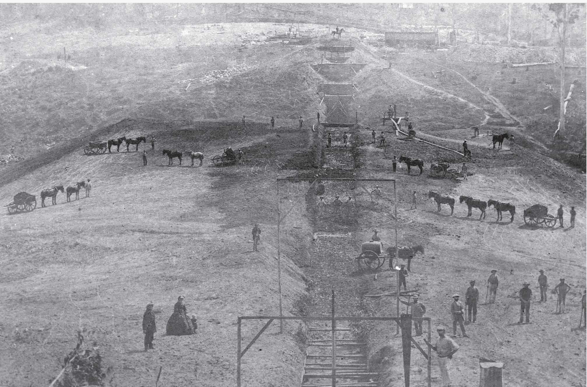
Dam Construction Puddle Trench. Workers constructing the Enoggera Reservoir, Brisbane, ca. 1864. Photo: John Oxley Library, State Library of Queensland
