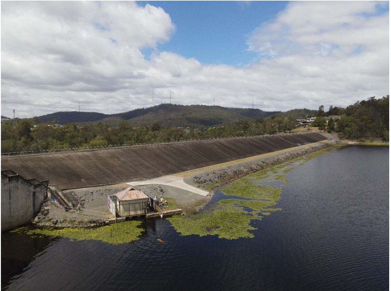
Valve House Note three inlet ports at water level Photo: Kyler Coghlan 2021
