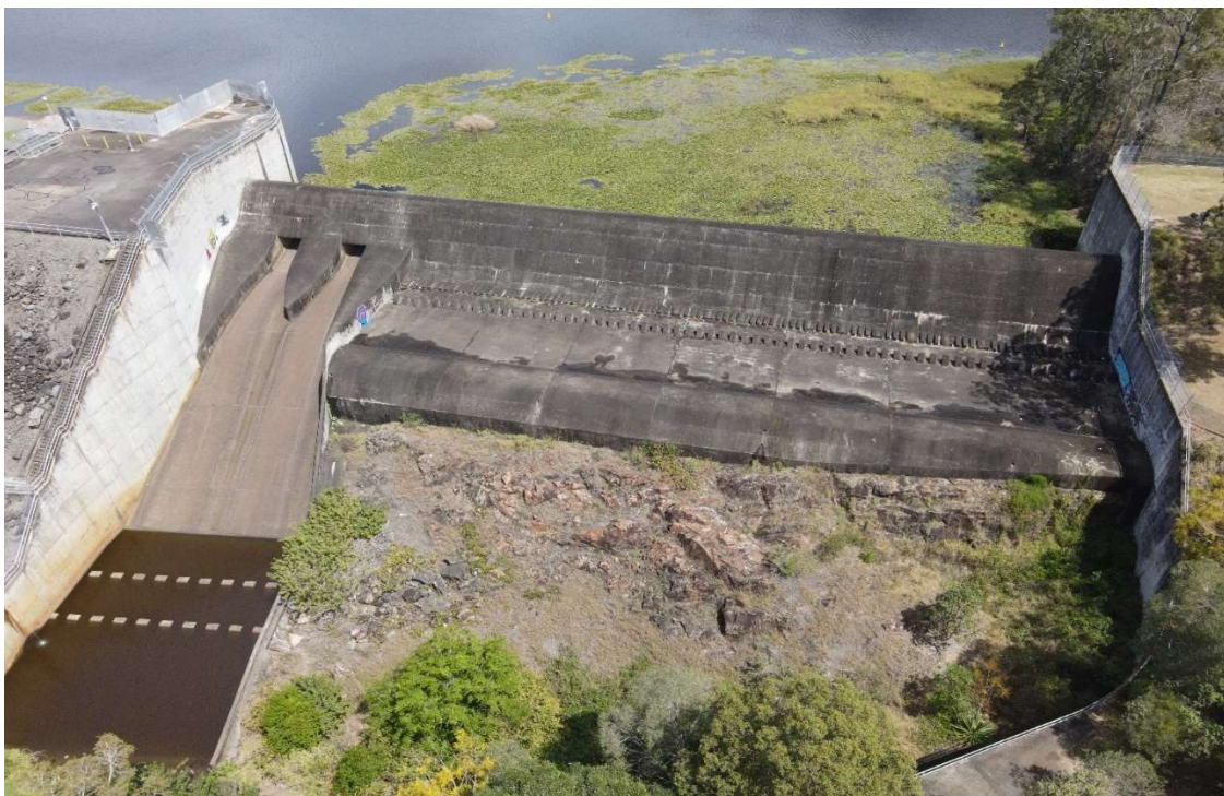
1976 Spillway – note outlets for low level flows
