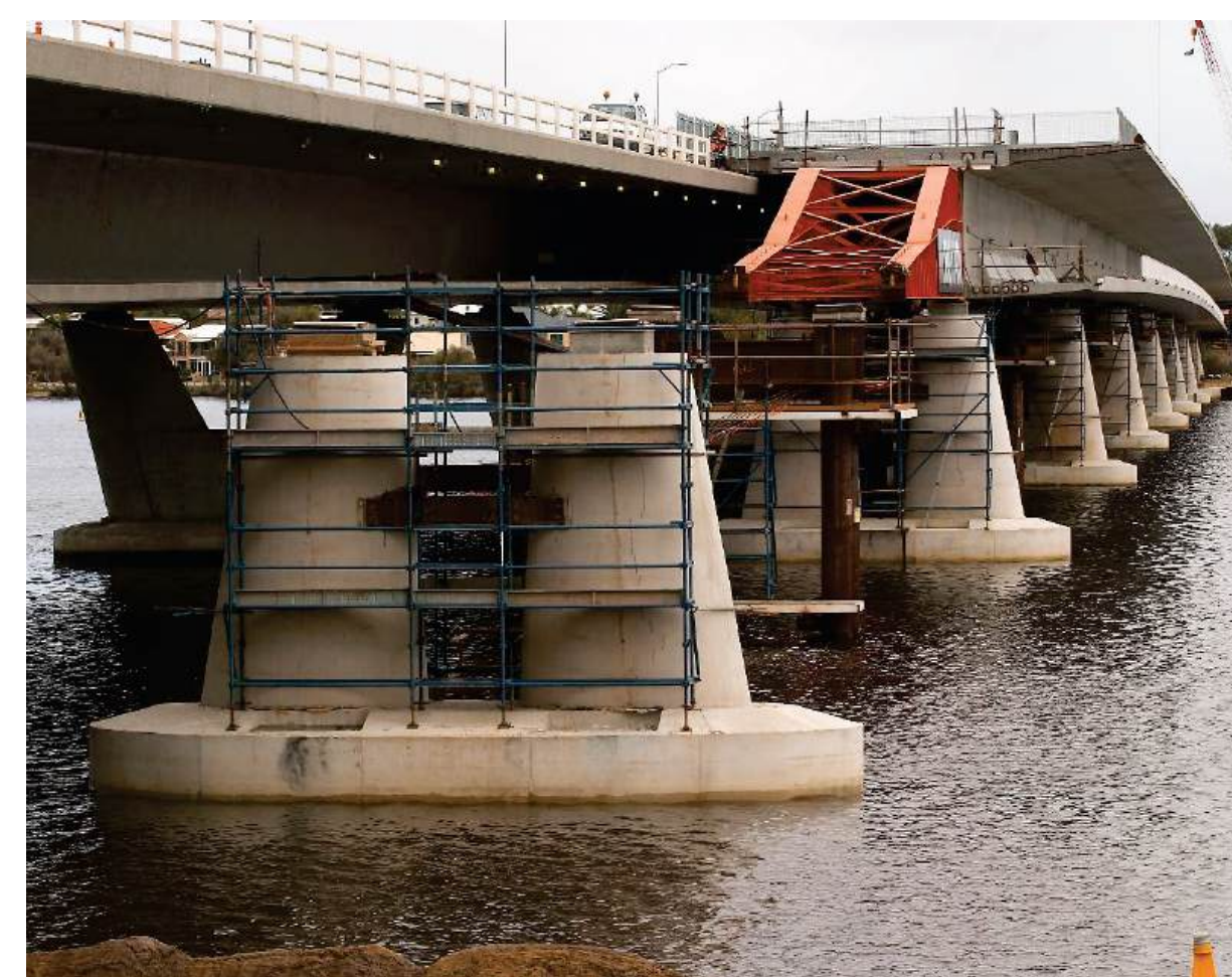
Launching of the 2007 Bridge
