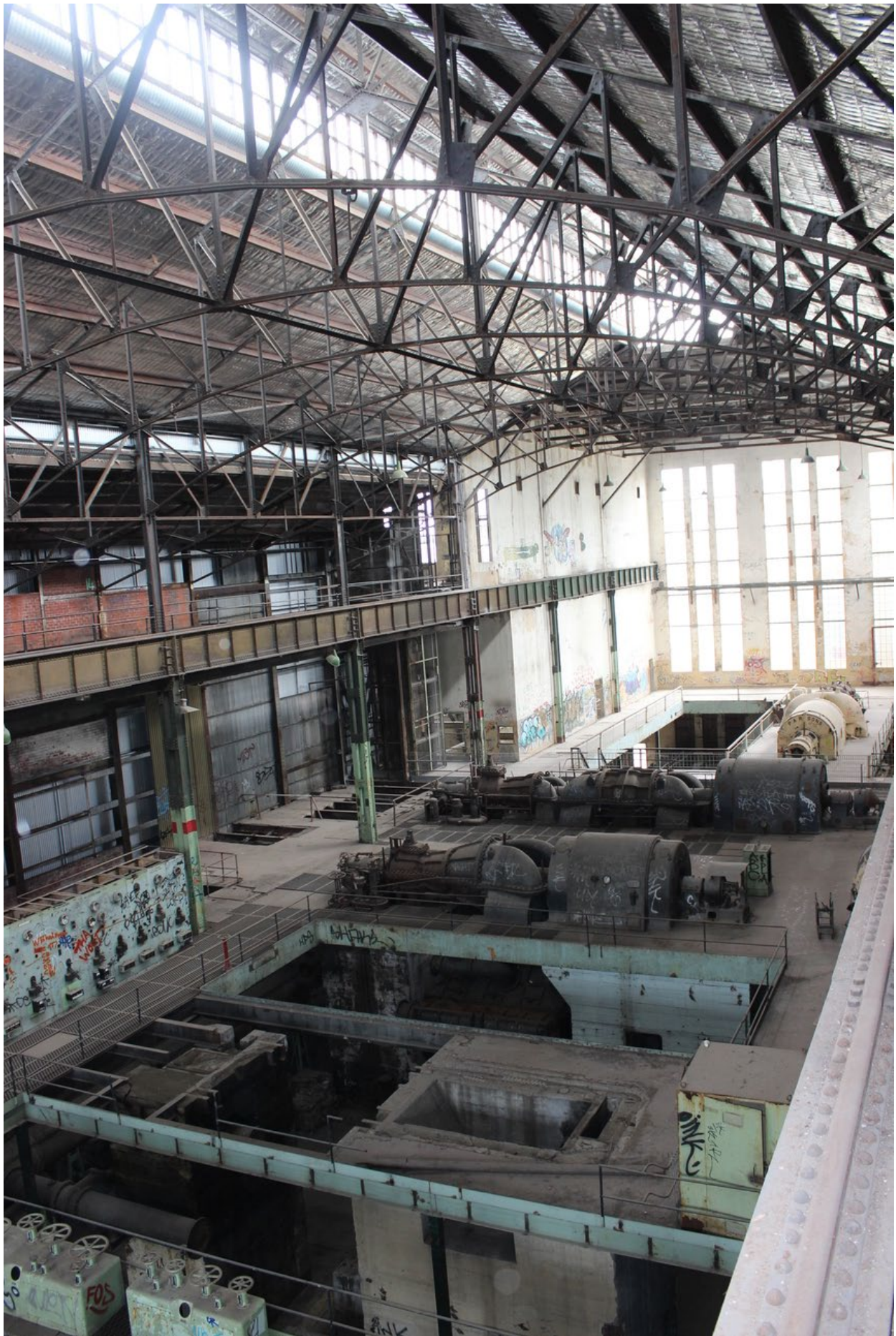
Figure 47: : Turboalternators Nos 4, 5 and 6
