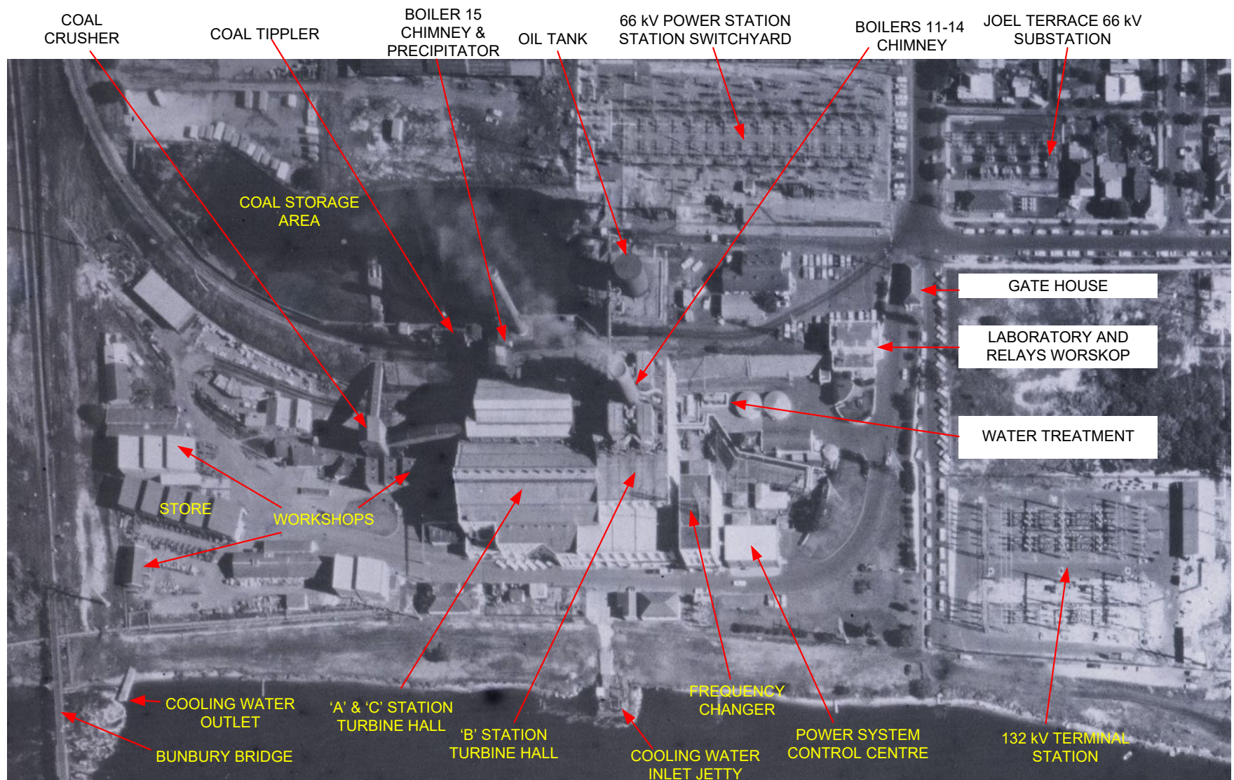
Figure 40: East Perth Power Station around the time of its Ultimate Development [Birds eye view]
