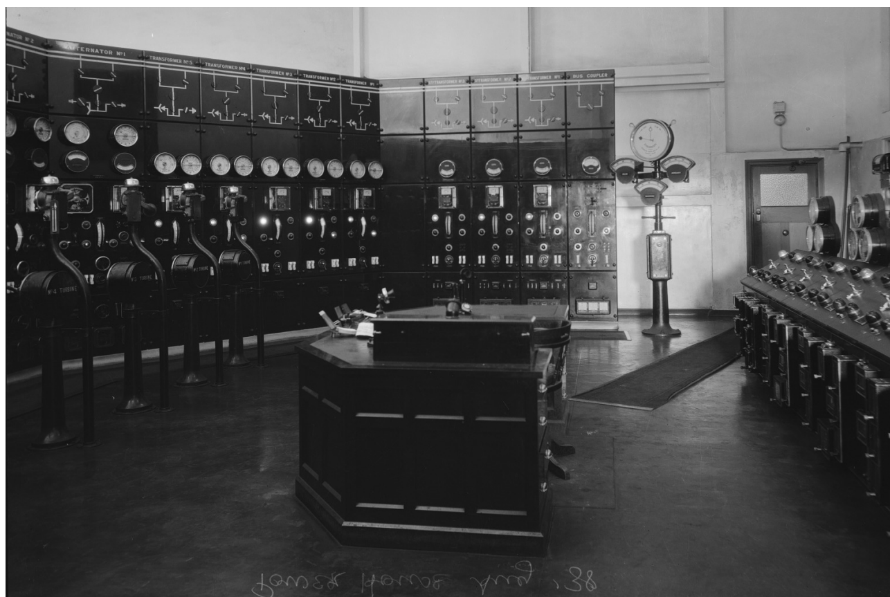
Figure 27: slwa_b2404120_2 Ctrl Room Aug 1938
