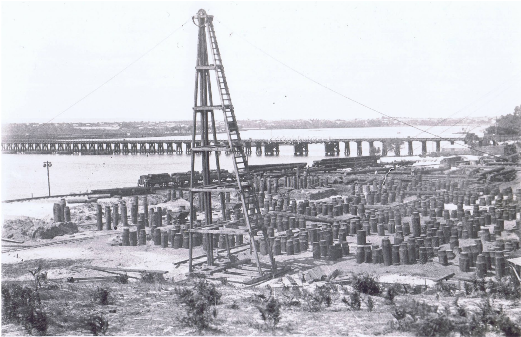
Figure 1: East Perth Power Station Ground Works circa 1914 [Plate 3]
