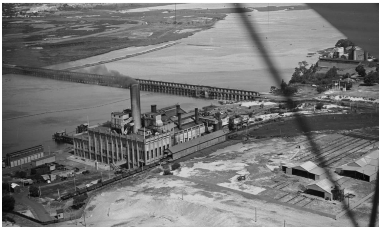
Figure 26: East Perth Power Station with only 3 of the 4 'B' Station Boilers installed. Not earlier than 1939. [call no BA575_295]
