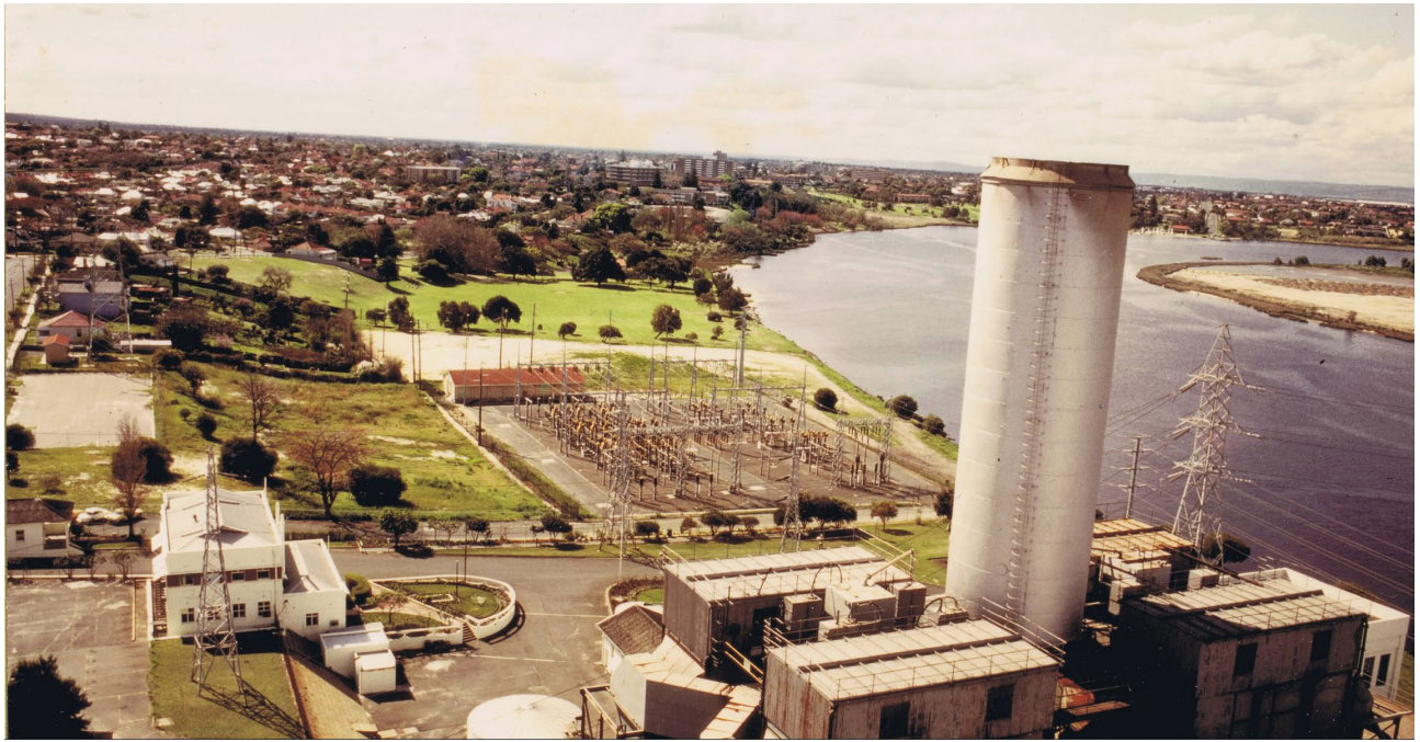
Figure 29: 'B' Station Precipitators viewed from 'C' Station Chimney [Plate 26]
