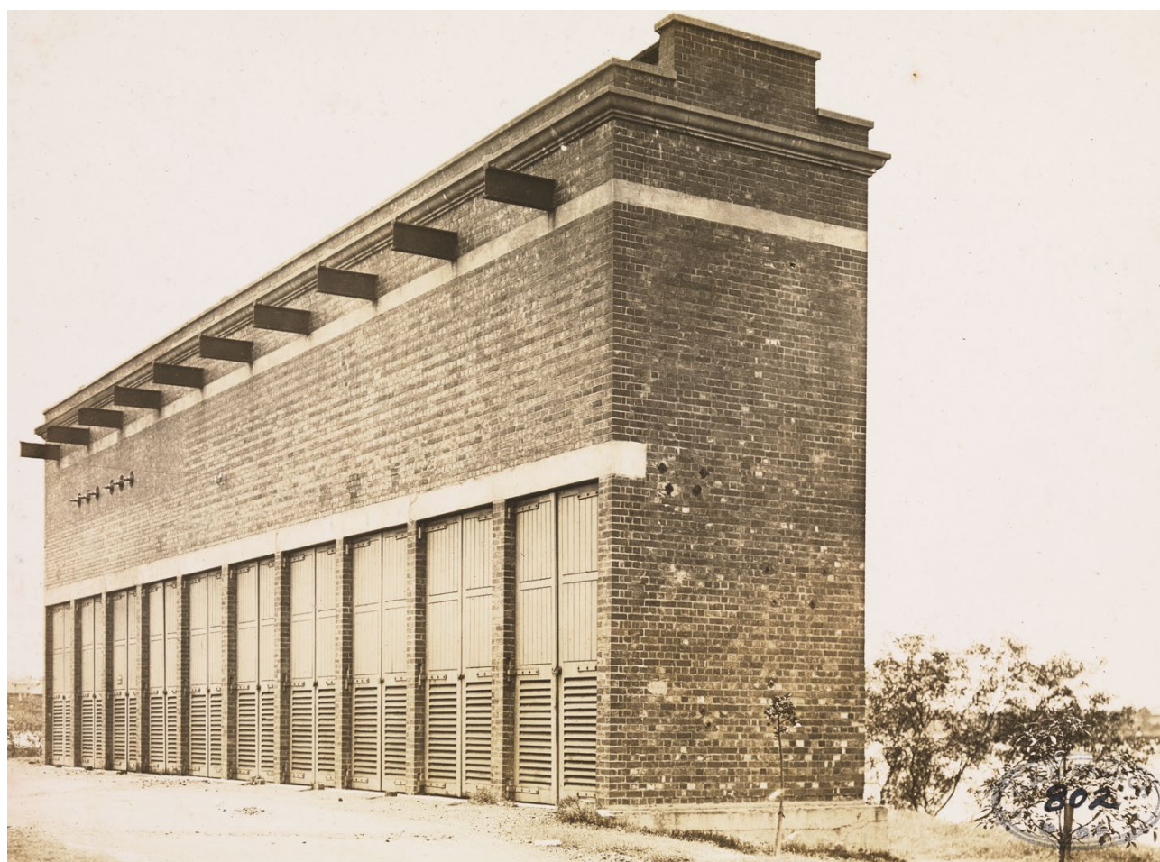
Figure 18: 6/20 kV step-up transformer building [BA2580 album 10]
