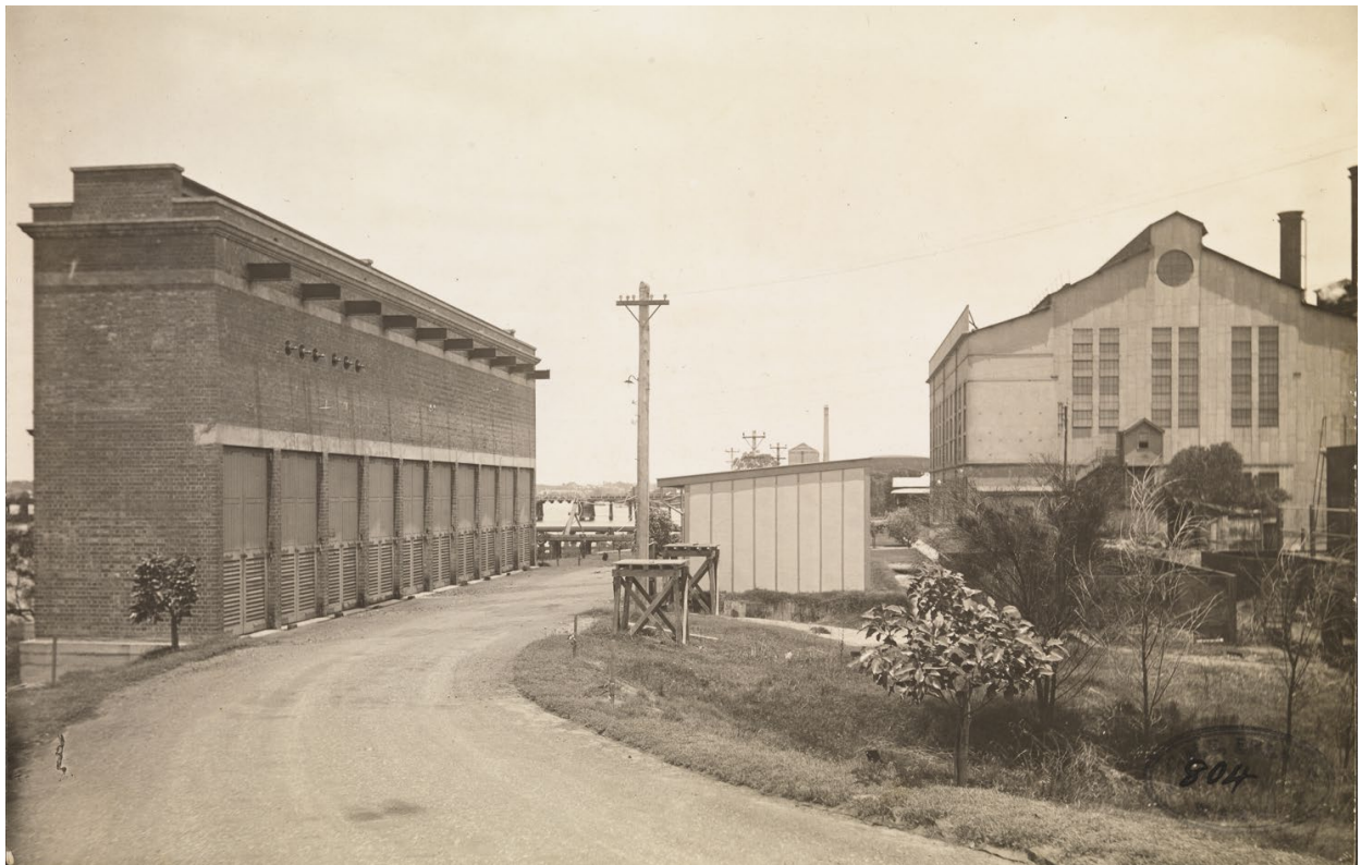
Figure 9: Step Up Transformer House – Reyrolle Switch House – Turbine Hall [BA2850 album 01]
