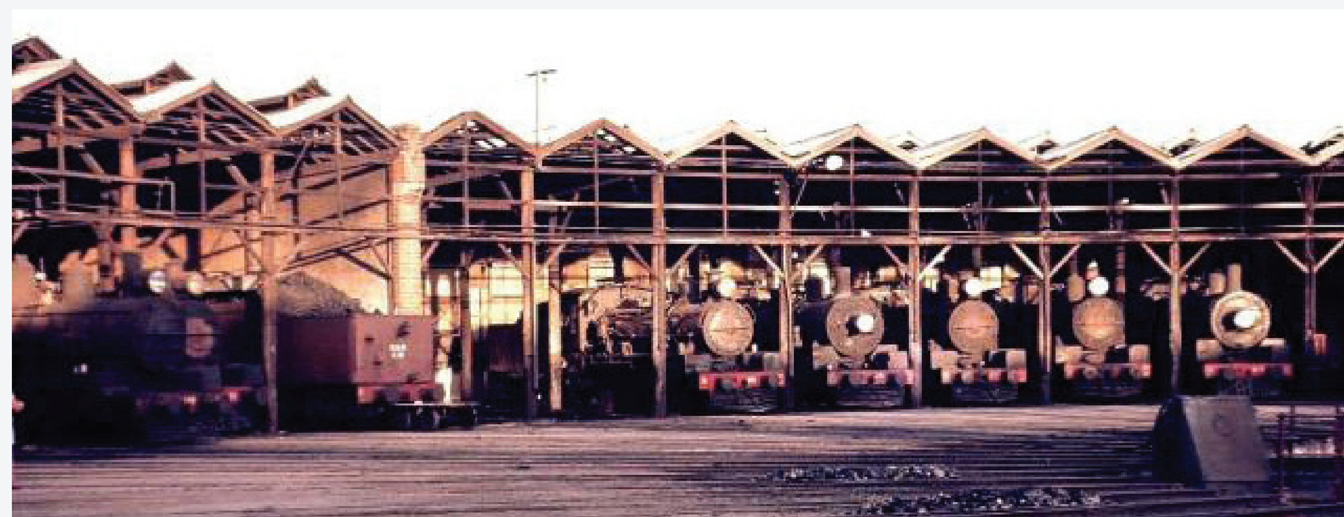
Ten of the 52 service bays with locomotives undergoing maintenance
