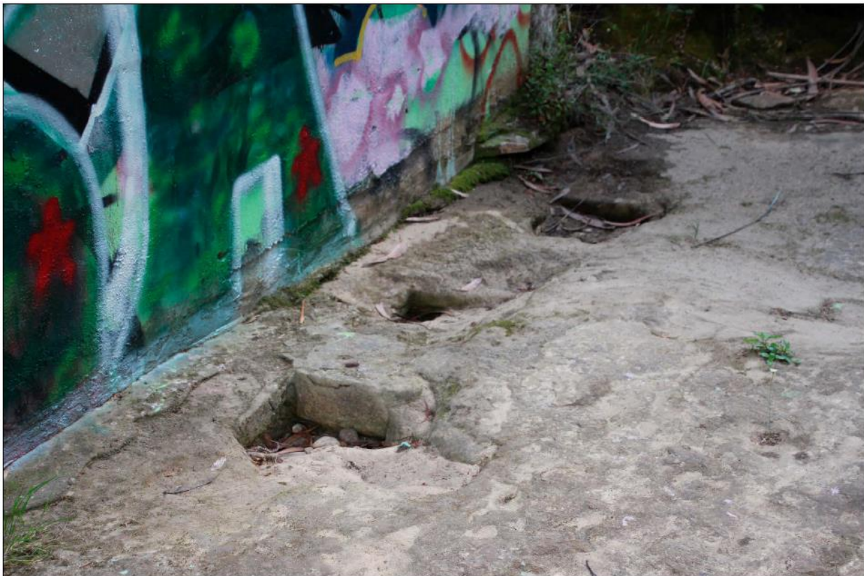
Figure 10. Timber Centering foundations, squared holes in bedrock beneath the arch (extract from CMP, photo Sid French)
