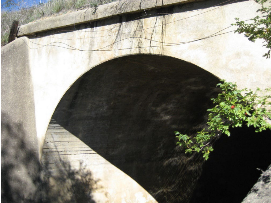
Figure 4 Eastern face of the Waterhole Creek Bridge with impressions of the formwork on the soffit. Stephen Buck 2007
