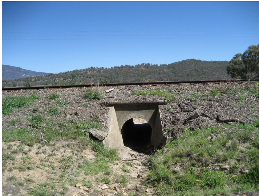
Figure 3A concrete culvert at 217 miles 6 chains. The location is stamped on the face wall of the culvert and corresponds exactly to the Working Plan. Stephen Buck 2007
