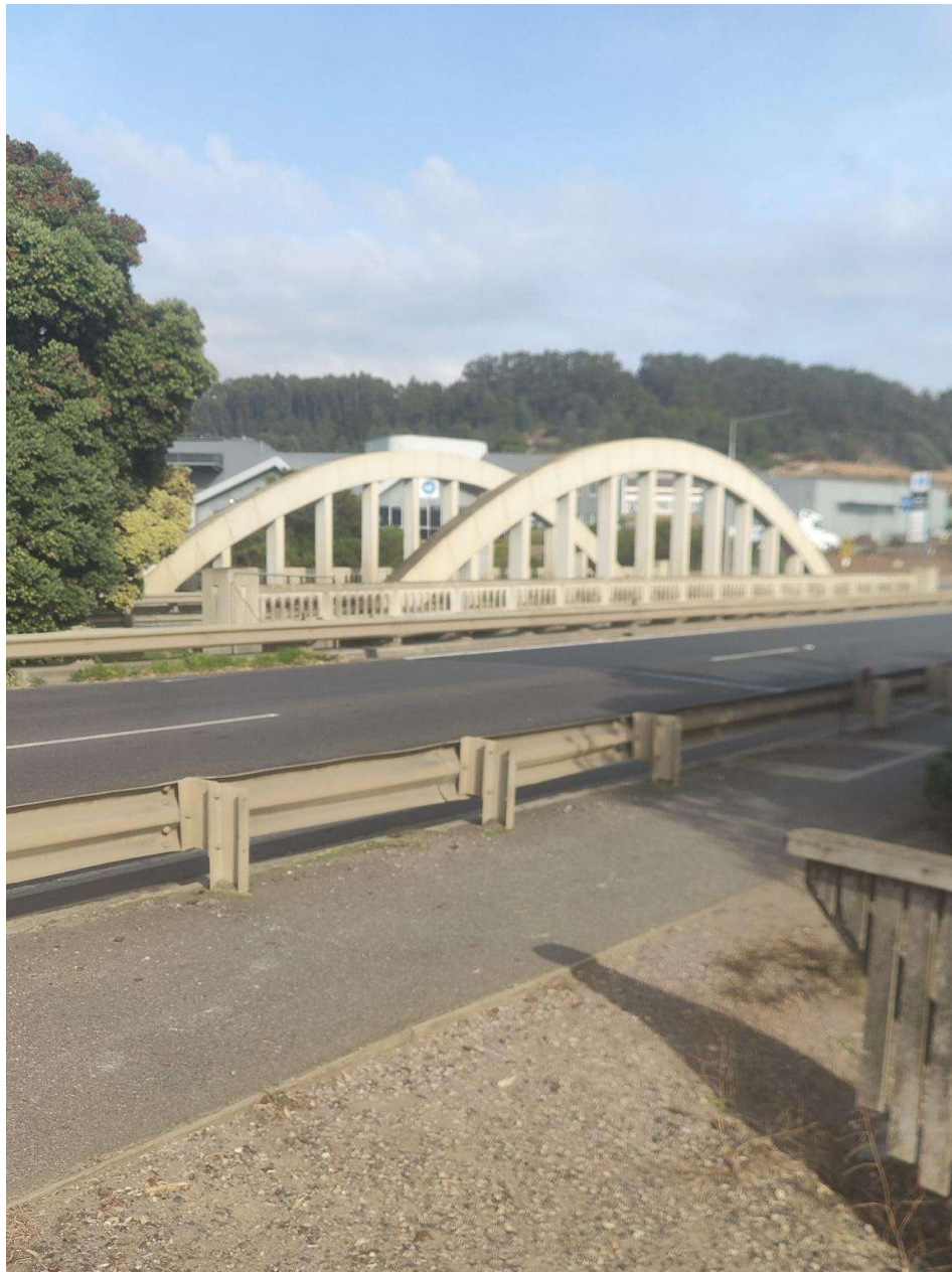
Photo 2: Northern elevation of bowstring arches (Photograph from Indrek Tults)
