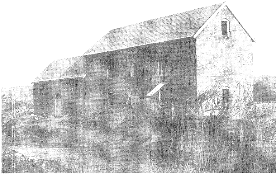
Fig. 2: Thorpe Watermill during restoration in 1975. This view is of the eastern side of the building and shows the redug head-race and the new roof. Photograph by Peter Bignell.
