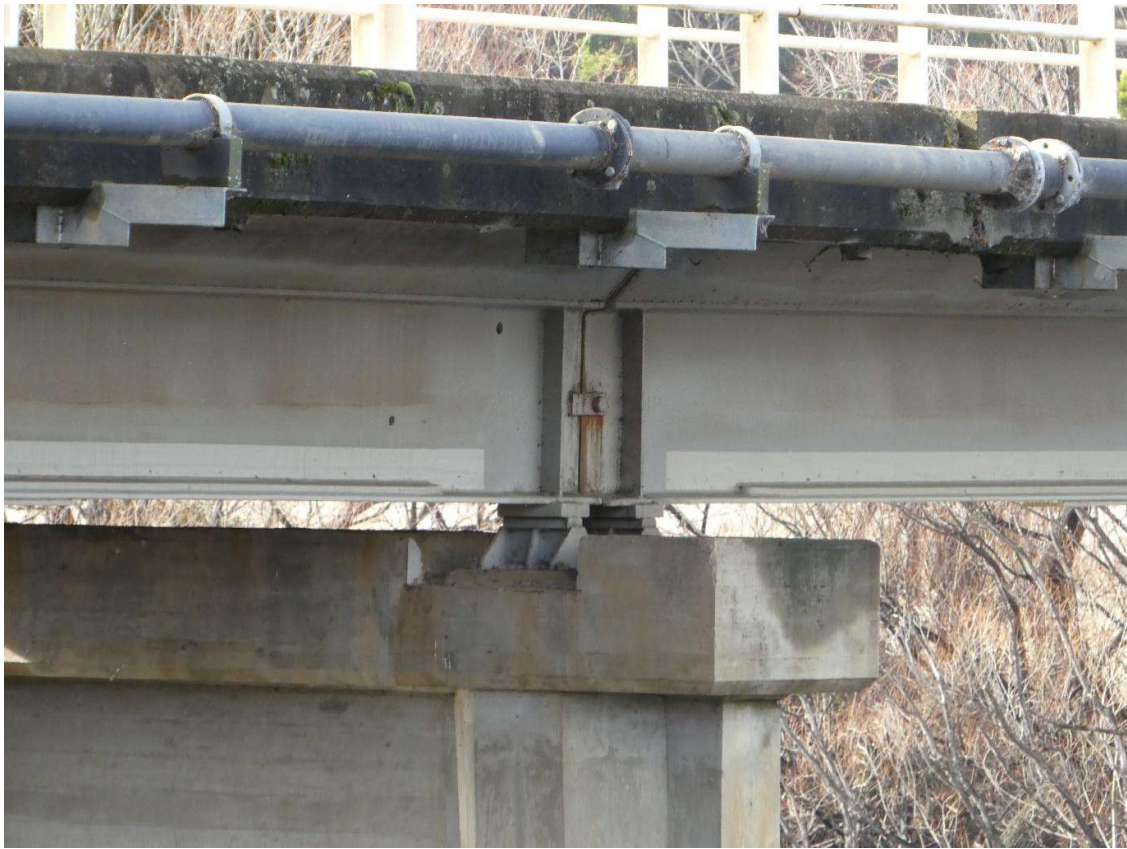
Photo 3: Detail of girder bearings and pier crosshead (Photograph taken by Graeme Nichols)
