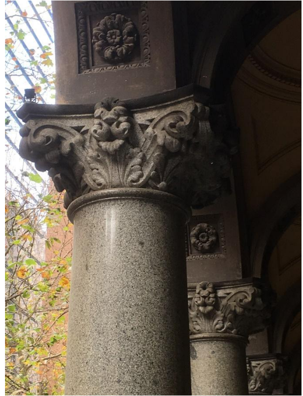
Moruya granite column
