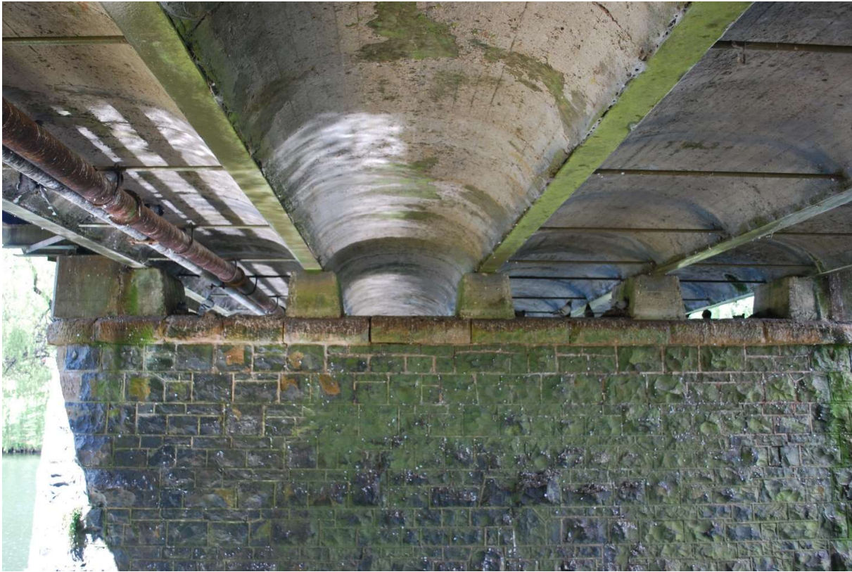
Photo 1: Photograph of the underside of the superstructure showing the concrete jack arches supported by steel beams (photograph taken by Graeme Nichols)
