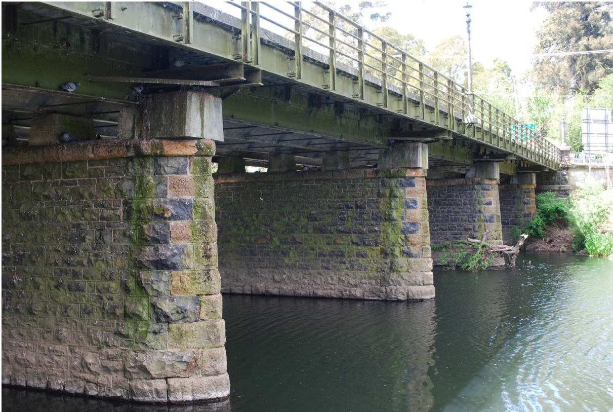
Photo 3: Upstream elevation of the bridge showing bridge widening (photograph taken by Graeme Nichols)
